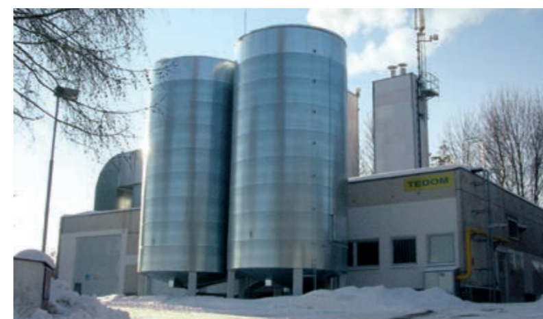
District Heating Plant, Světlá n. Sázavou, Czech Republic
